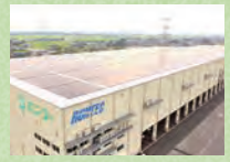
Installing solar power and energy-saving equipment at PD centers
