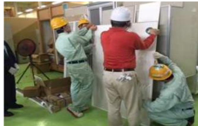
Installment of prefabricated bathtub units
