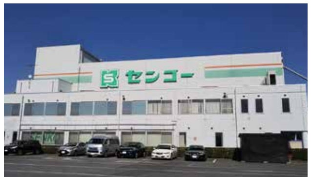
The existing Ibaraki PD Center switched over to 100% LED lighting
