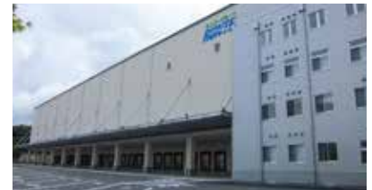
Runtec's Kansai Branch opened in July 2019 (SENKO Group's first large generation and on-site consumption)
