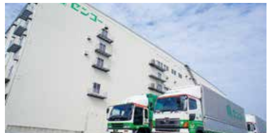
Urawa PD Center achieved 100% LED lighting by utilizing subsidies
