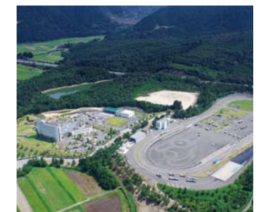
Crefeel Koto, opened in 1996, is a distribution and traffic safety education and training center offering hands-on experience that covers a total of 270,000 square meters
