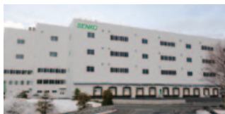
Sapporo PD Center No. 2 Warehouse
