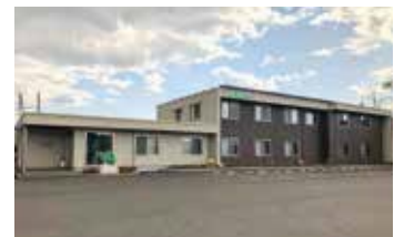
March 2018, Senko Co., Ltd. Ibaraki Housing Branch
