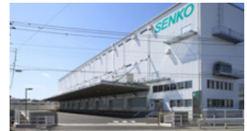
Higashi Fuji PD Center (started operation in April 2018, began operating solar power plant in December 2018)
