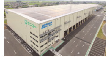
Kazo PD Center warehouse No.2 (started operation in August 2018)
