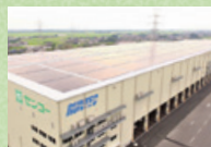
Installing solar power generation / energy-saving equipment at PD Centers
