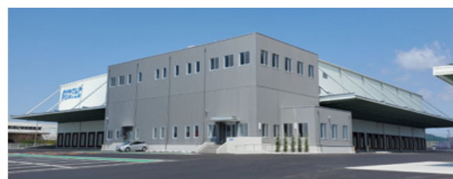
Runtec Corporation's Moji Branch, which began operations in April 2020
